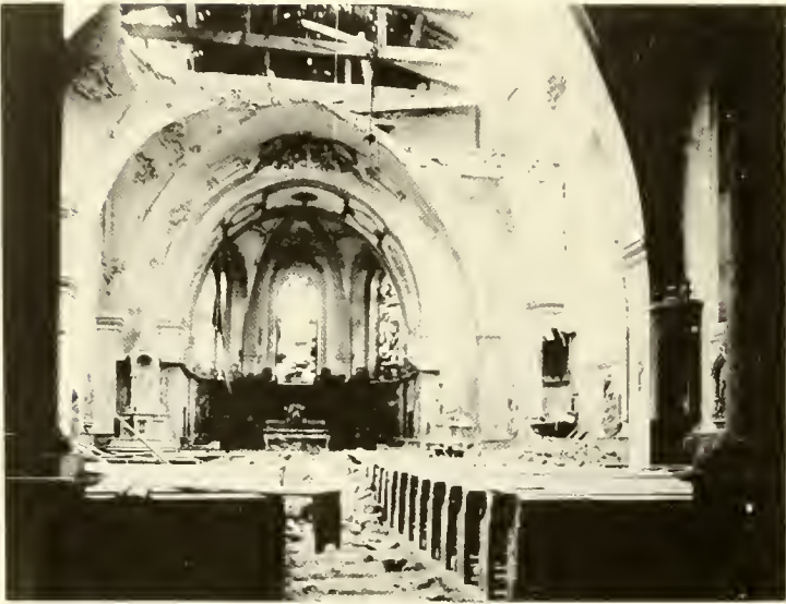
Interior of THAUCOURT Church
